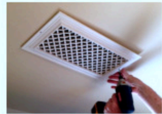
Install the new grill
