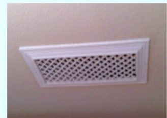
Ready for paint, well worth the extra steps
