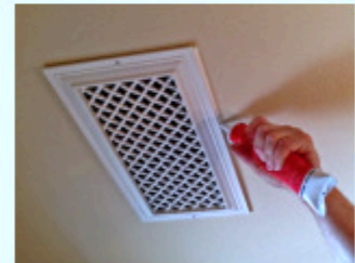
Caulking seam with latex caulking
